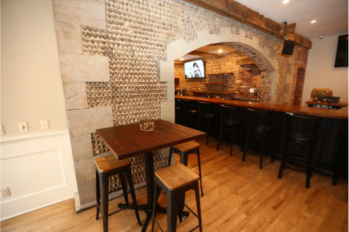
Over the bar, you can see the exposed original cobblestone wall from 1844 that has been preserved. (John Hickey/Buffalo News)
